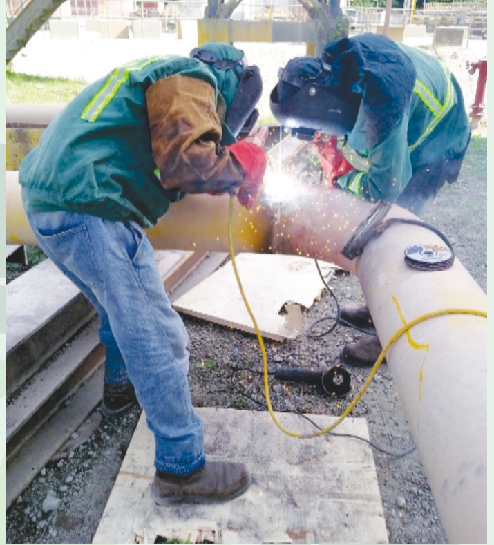
Welding of 10 Inches pipe at Lafarge Mfamosing Plant, Calabar
