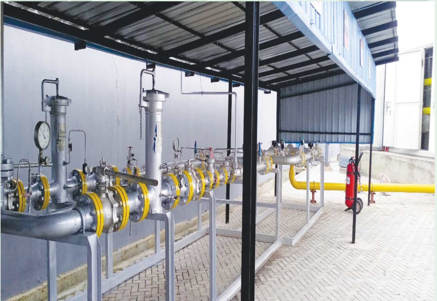
Fabrication and Installation of Pressure Reduction and Metering Station at GASCO Marine, Abeokuta
