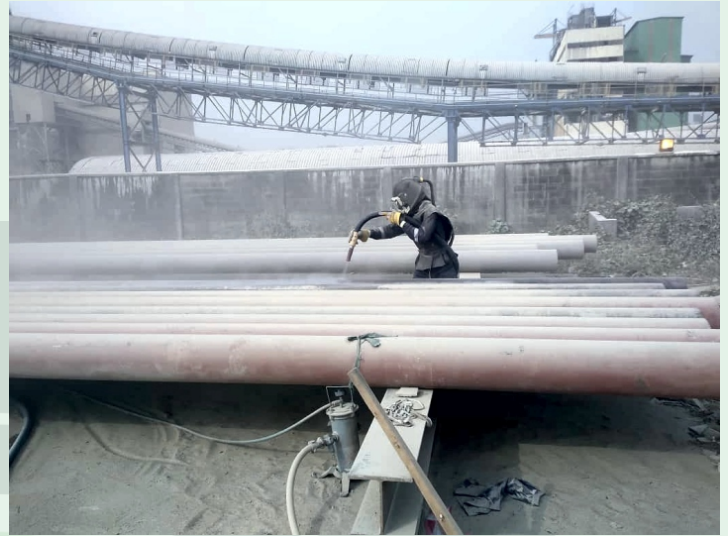
Sand Blasting of Pipe at Lafarge Mfamosing Plant, Calabar.
