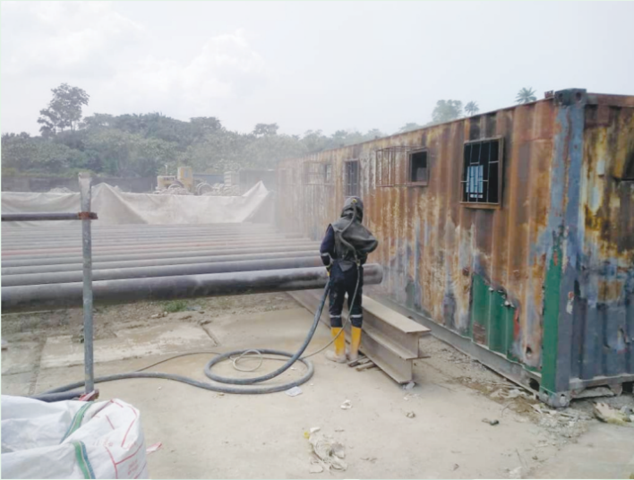
Sand Blasting of Pipe at Lafarge Mfamosing Plant, Calabar.
