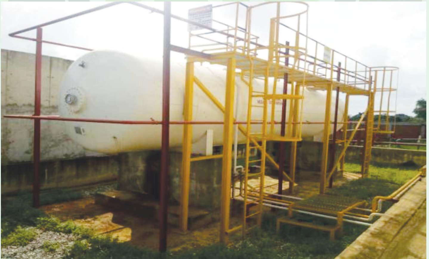
Installation & Construction of LPG Storage tank foundation and Containment wall at NAMPK.
