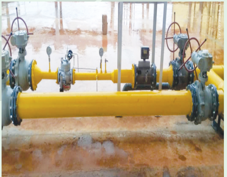
Installation of Aperva Regulator at Ropes and Belt Itori, Ogun State
