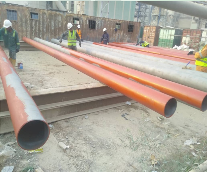
Painting of Sand blasted pipe with Red oxide
