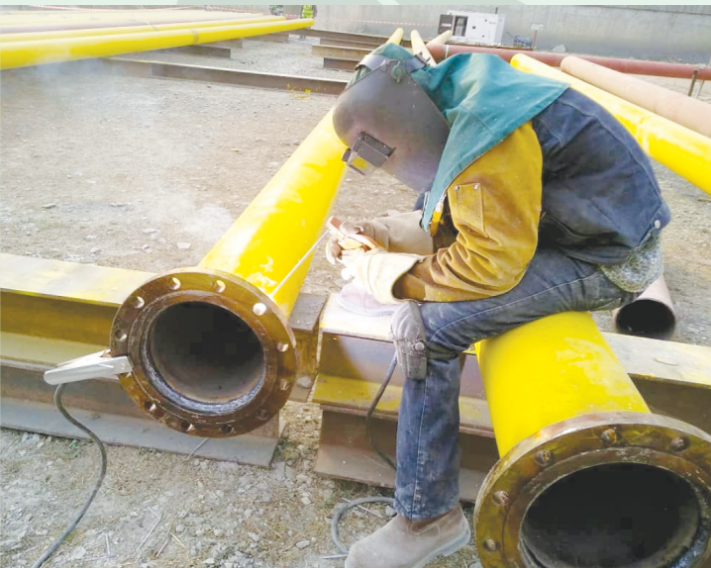
Welding of 10" pipe & Flange @ Lafarge
