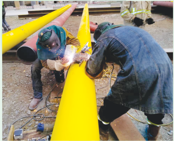
Joining of two 10" pipe together @ Lafarge, Calabar
