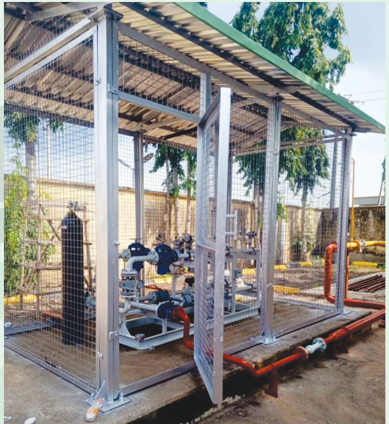
Fabrication and Installation of Dual streams PRMS (0.8 SCM) for Nature Bounty Foods, Abeokuta
