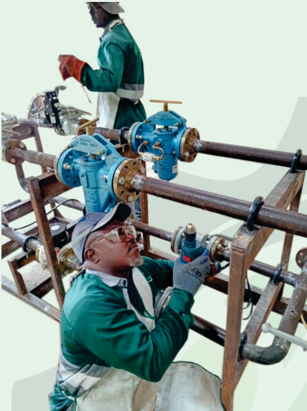
Fabrication and Installation of Dual streams PRMS (0.8 SCM) for Nature Bounty Foods, Abeokuta
