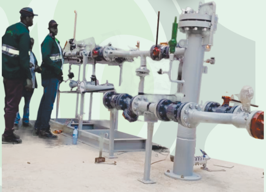
Fabrication and Installation of Dual Stream PRMS (1MMSCM) for ENTEC
